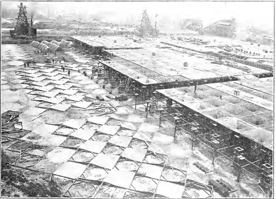
FILTER BEDS Pittsburgh Filtration Plant
